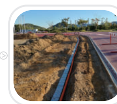
Construction of rainwater saving tank *Option: Rainwater saving tank
