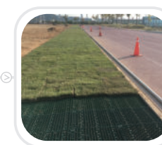
Installation of natural grass and grass protection mat
