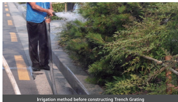
Irrigation method before constructing Trench Grating
