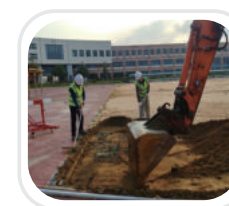
Levelling of the surface.
